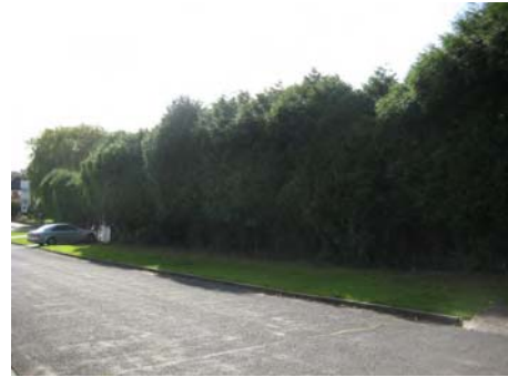
Picture 4.100 Boundary treatment to 2 Valencia Road on the upper Kerry Avenue side is typical of the taller, hedges here that form boundary treatments
