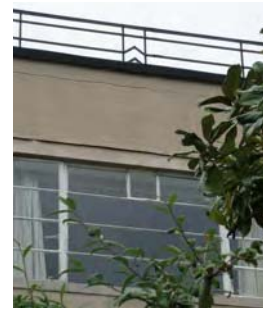
Picture 4.46 Good arrow detail within railings of 4 Valencia Road
