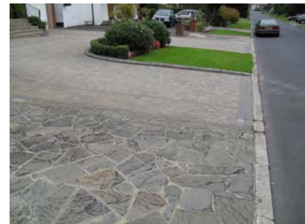
Picture 4.108 Excessive hardsurfacing introduces a barren appearance at odds with the intended design of the CA
