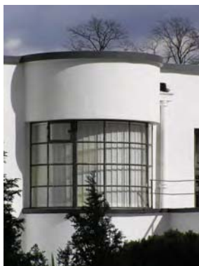
Picture 4.82 Original windows complement the strong geometrical design of the building
