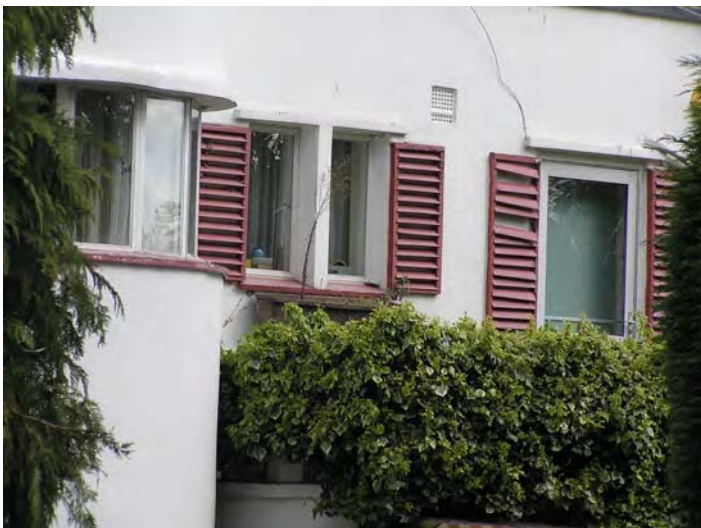
Picture 4.85 Original shutters on number 4 Kerry Avenue
