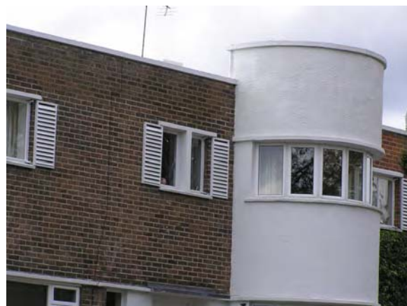
Picture 4.86 Original shutters on 3 Kerry Avenue complement the Modernist Design
