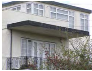
Picture 4.48 First floor balcony to 8 Valencia Road
