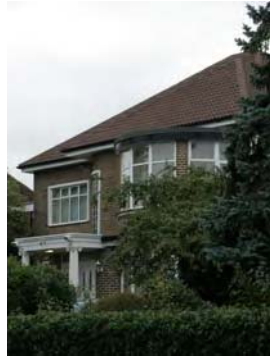
Picture 4.51 14 Valencia Road, just outside the CA - originally constructed in Modernist design
