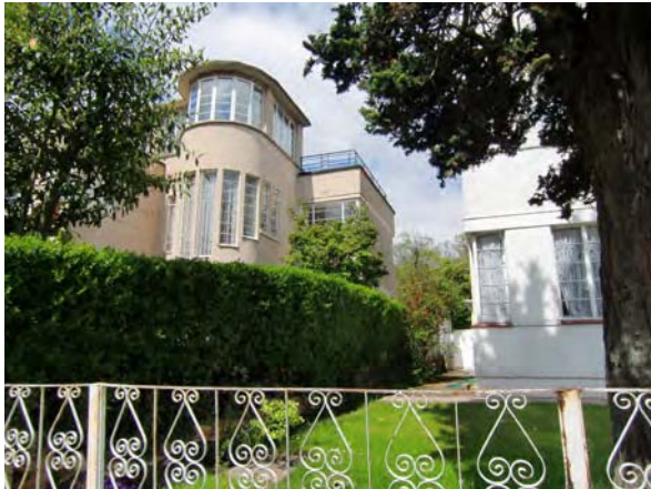
Picture 4.24 2 and 4 Valencia Road - Vertical emphasis to these buildings
