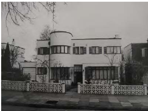
Picture 4.59 Number 4 Kerry Avenue before some of the modern alterations to the building (date of the photo unknown). Source: Local history library
