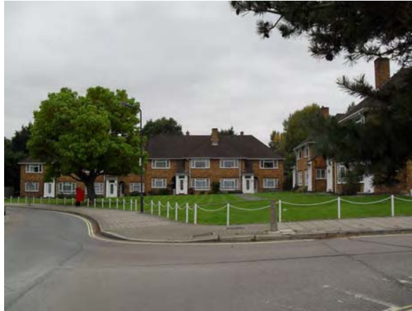
Picture 4.15 Part of the formally planned semi-circular opening to the CA, lined by white posts
