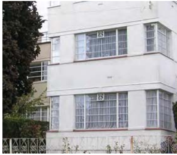
Picture 4.45 Good arrow detail within window of 2 Valencia Road
