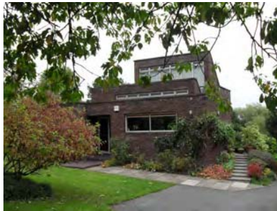
Picture 4.68 Locally listed 16 Kerry Avenue - a good example of late Modernist architecture
